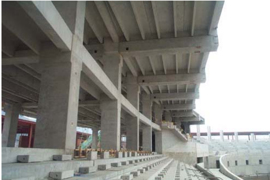
Fig. 7 Long Cantilever beam constructed
